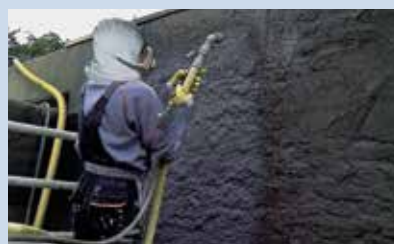
Reprofilage des supports
